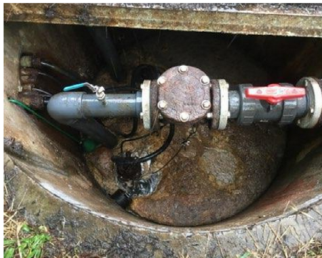
Figure 5. Total mat coverage in shallow wet well lift station #15.5.
